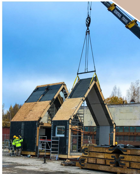
Delivery & Installation process
